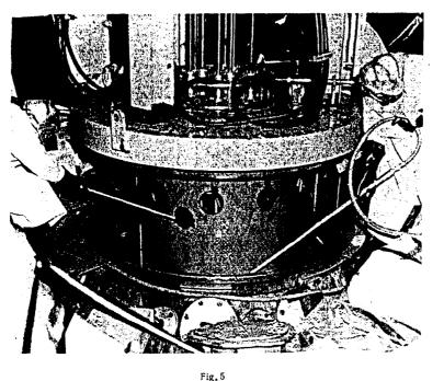
WTR reactor vessel head removal and decontamination
