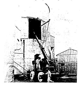
Fig. 20 Performing entry into the SL-1 reactor building
