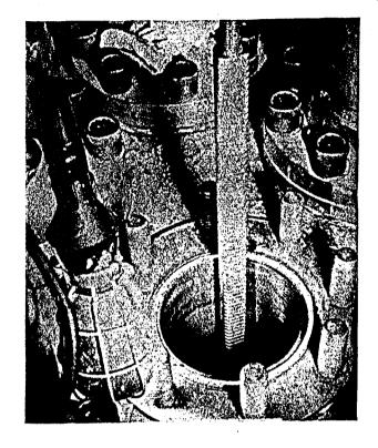
Fig.42 SL-1 control rod drive rack (pre-accident photo)
