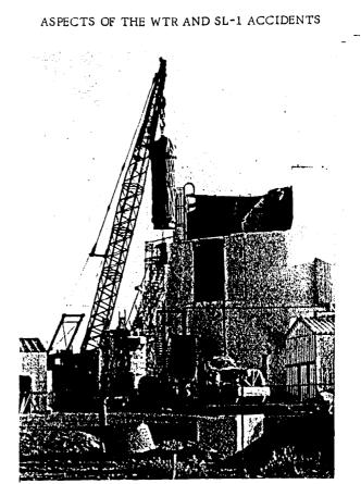
Fig.32 Pressure vessel being removed from SL-1 reactor building
